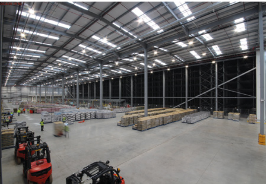
LDH Sproughton Warehouse, the automated warehouse built in Ipswich, UK.
